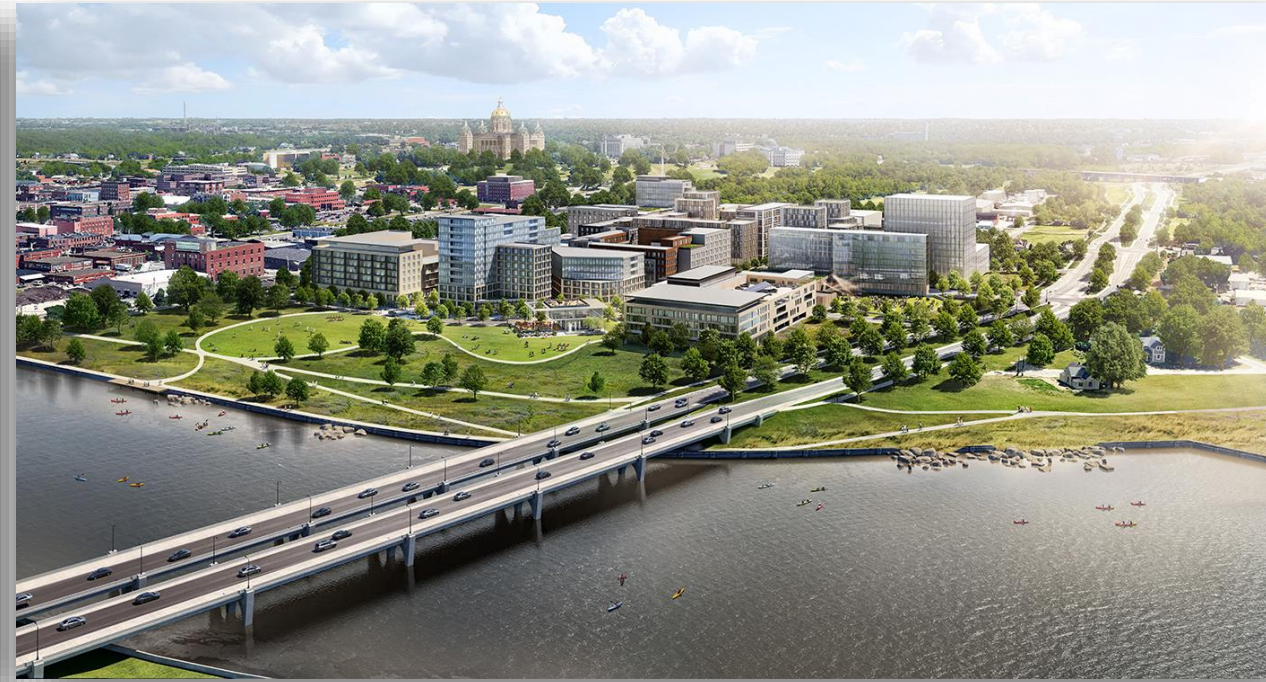
A rendering of the completed Market District redevelopment
