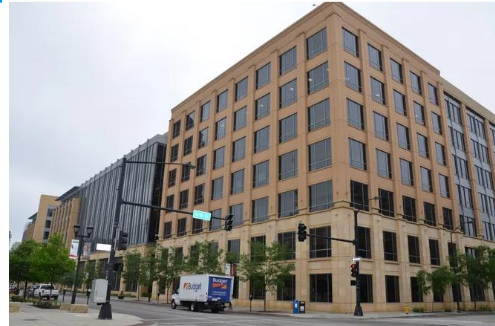
American Equity Life Holding Co. is moving from West Des Moines to this Nationwide Mutual Insurance building at 1100 Locust St. in West Des Moines. Polk County Assessor/Special To The Register
